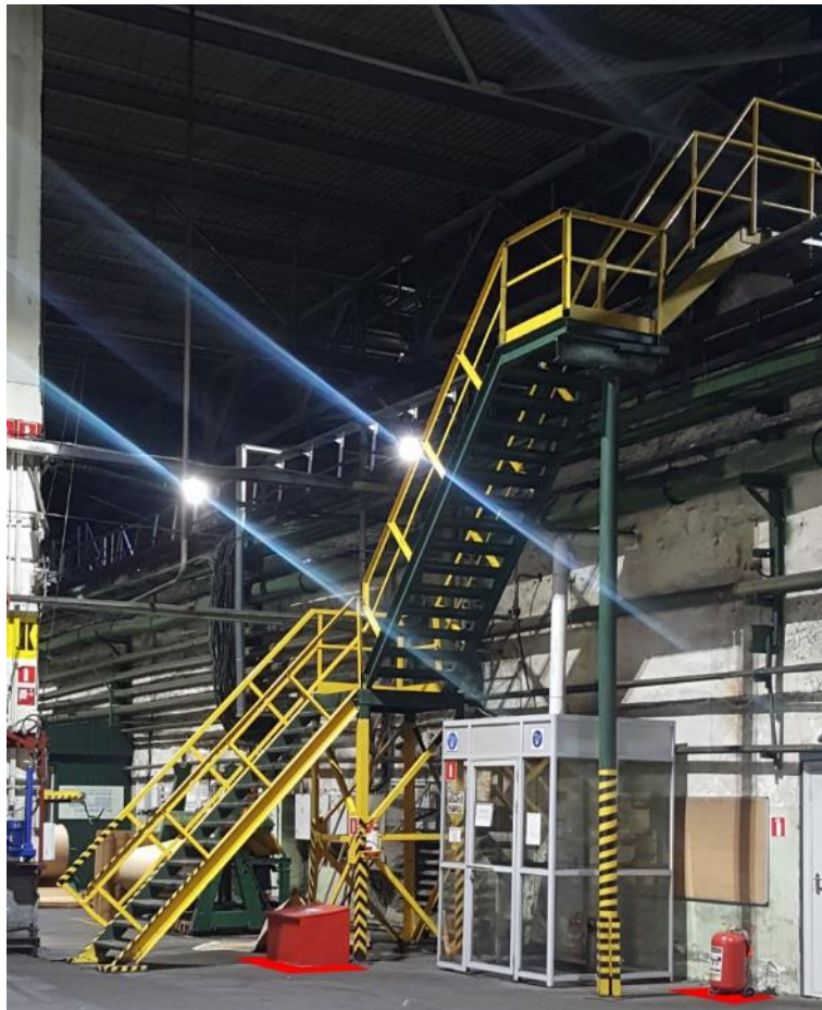
Figure 70 – sample designation of permanent barriers of stairs
