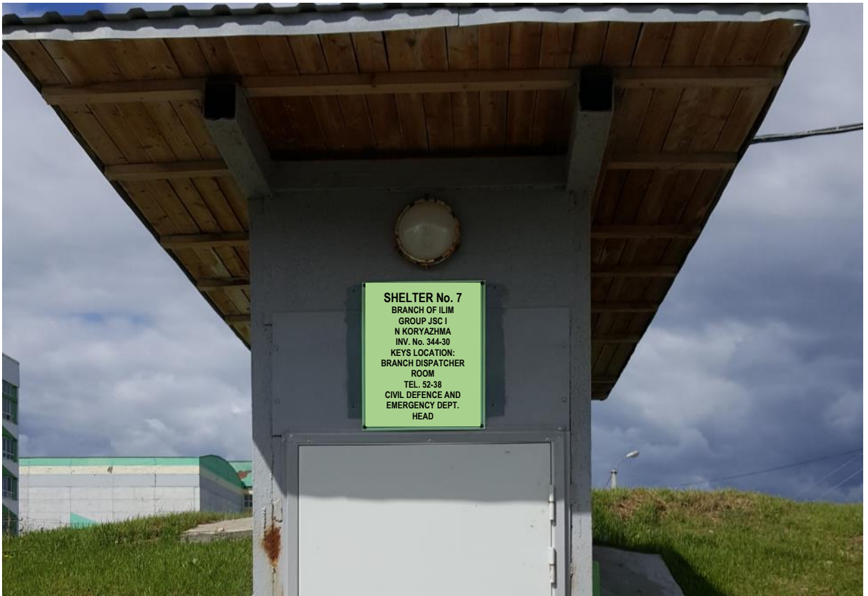
Figure 109 – sample information signboard of a civil defence shelter using photoluminescent materials
