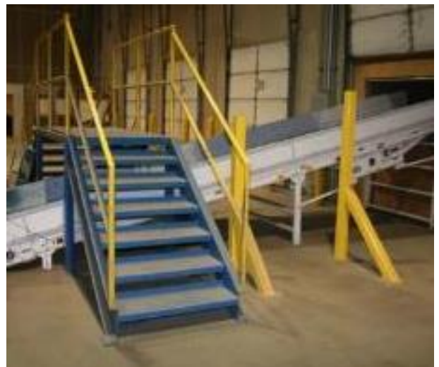
Figure 86 – sample crossing bridge
