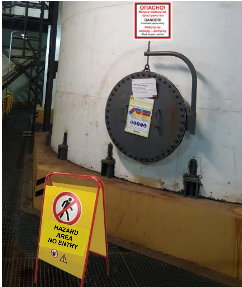
Figure 96 – sample stander installation at the hazard area boundary
