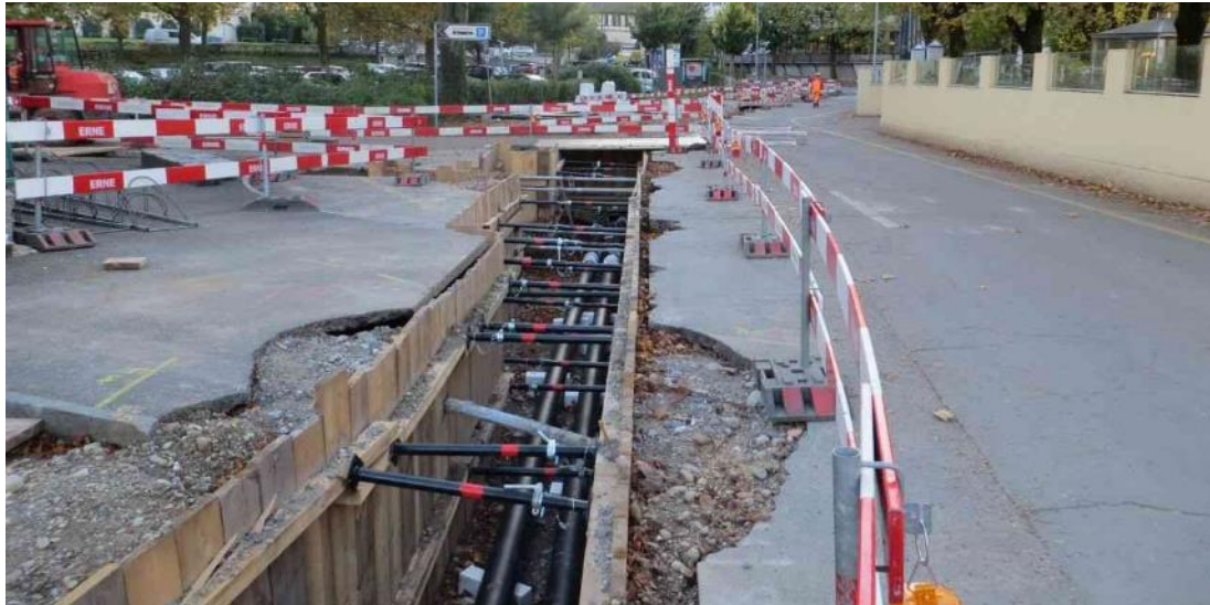
Figure 85 – sample enclosure of open trenches
