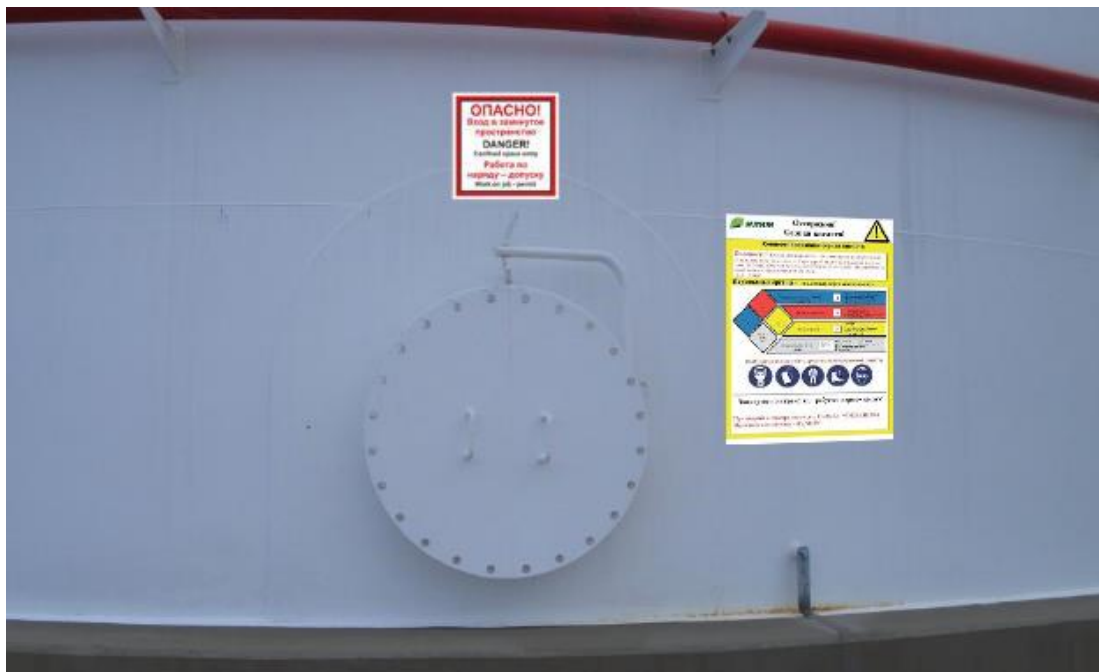
Figure 92 – sample placement of warning plate at the entrance to the confined space
