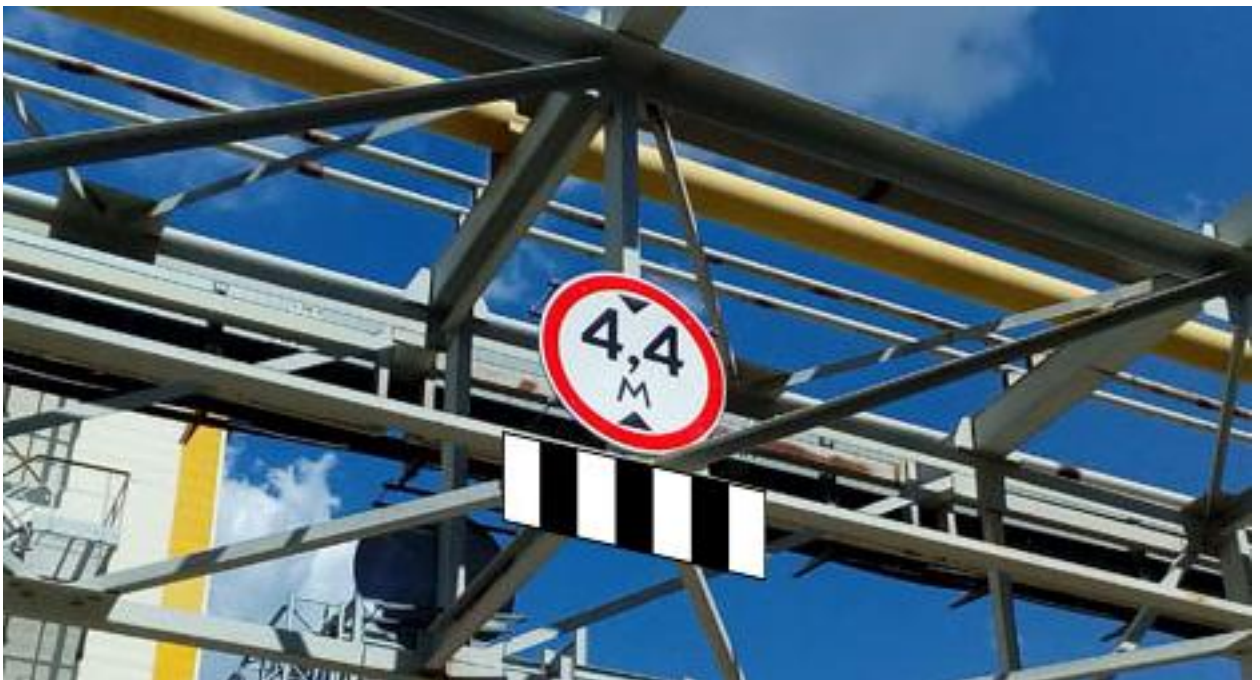
Figure 17 – sample “Height limit” sign installation
