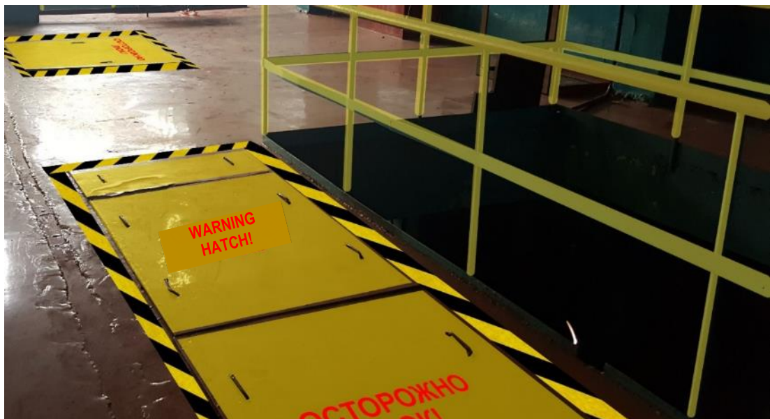
Figure 88 – sample painting of a process opening cover in the floor
