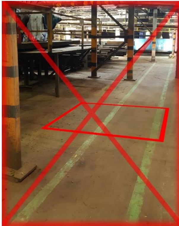
Figure 65 – sample unacceptable use of red floor marking
