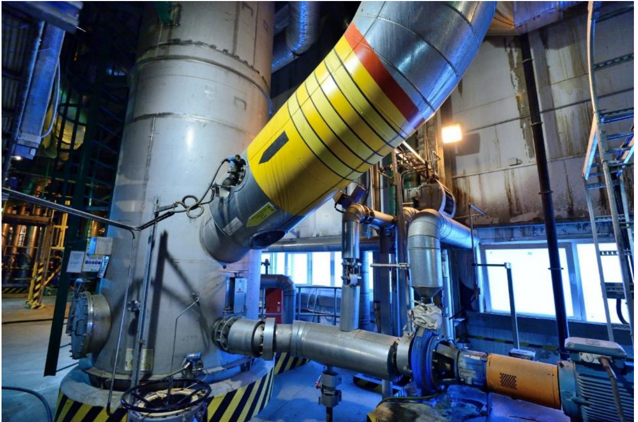
Figure 101 – sample painting with warning rings
