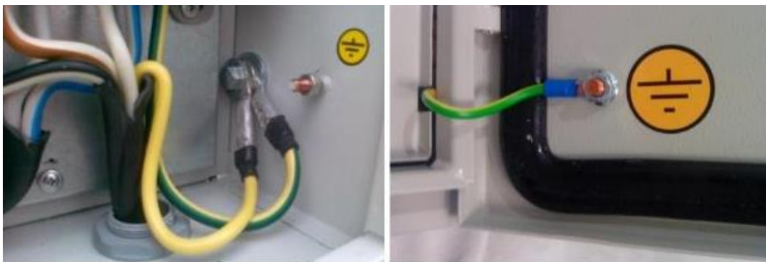
Figure 83 – sample placement of grounding sign
