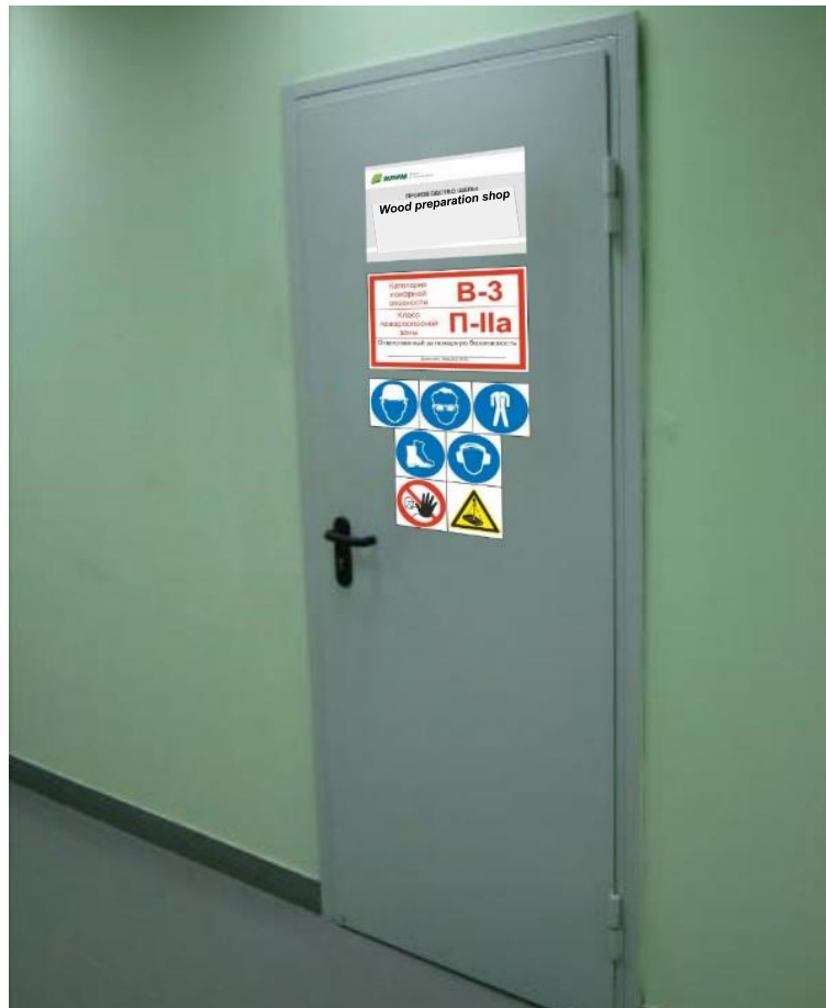
Figure 91 – sample placement of safety signs and information plates at the entrance to the production shop area
