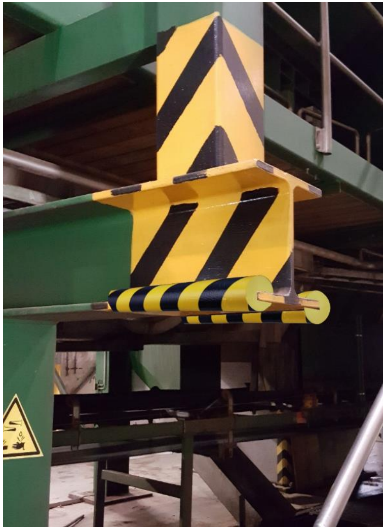
Figure 66 – sample designation of low beams
